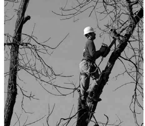
PVREA's arborists trim trees before they interfere with electric power lines.
